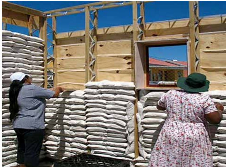
Insulation with sandbags, Princeton Technical High School.
